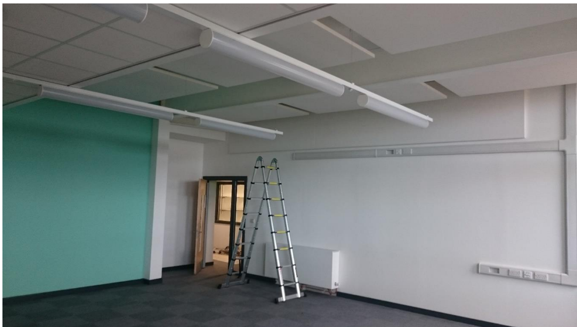
Figure 5: Typical primary classroom with bulkhead for ventilation unit, rafts and wall panels
